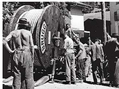
Laying of 420 kV oil-filled cables in Switzerland in the 1960s
