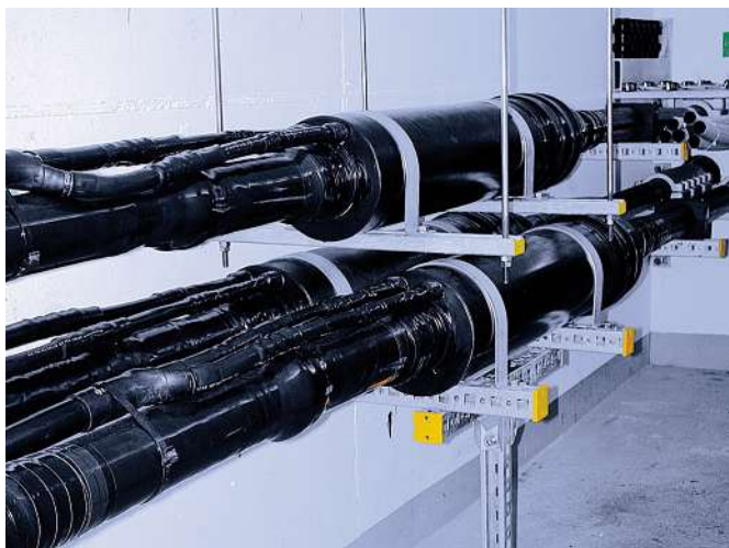
Joints with Cu-tube and HDPE coating in a concrete tunnel
