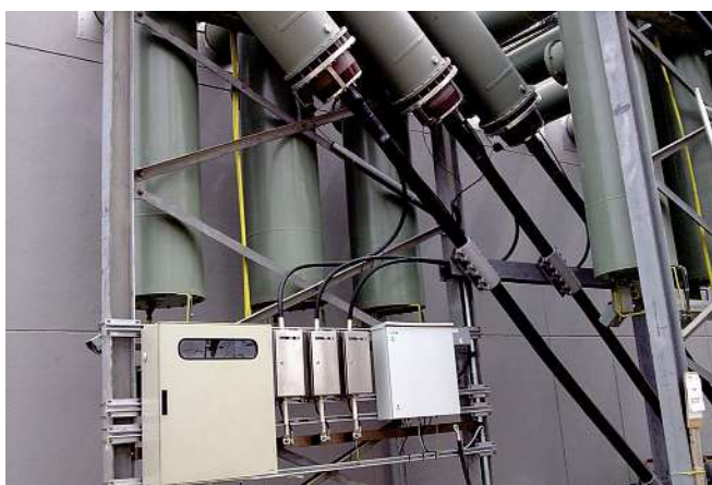
GIS-terminations of the highest voltage level (550 kV) in Egypt
