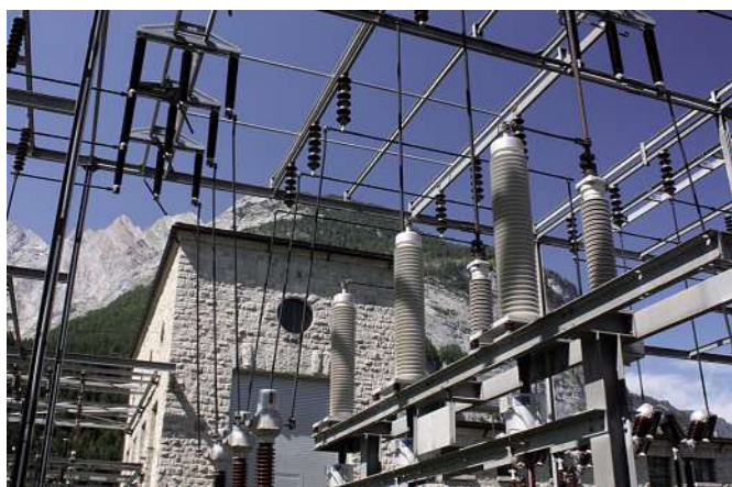
Outdoor terminations with composite insulators in Switzerland
