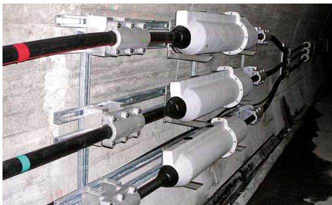
Joints with polyester protection box in a concrete tunnel
