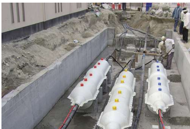
Installation of transition joints in Germany
