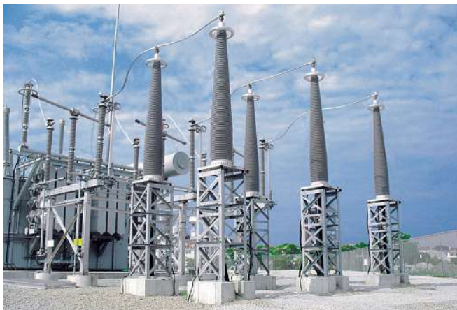
Outdoor terminations with porcelain insulators in the USA
