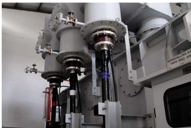
Transformer terminations in indoor application in South Africa
