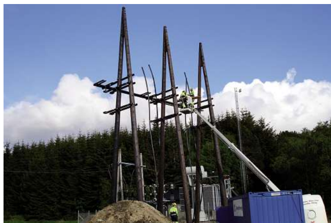
Preparation for the installation of outdoor terminations in Norway
