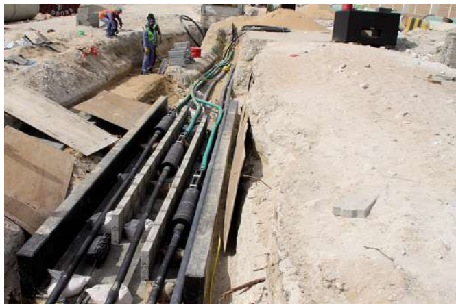
Installation of joints in Abu Dhabi
