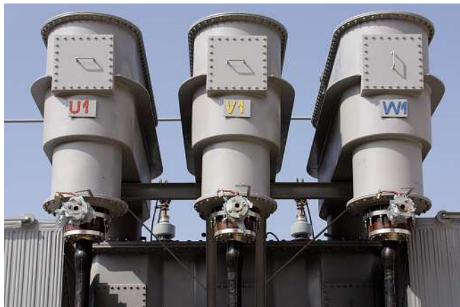
Transformer terminations in outdoor application in Jordan
