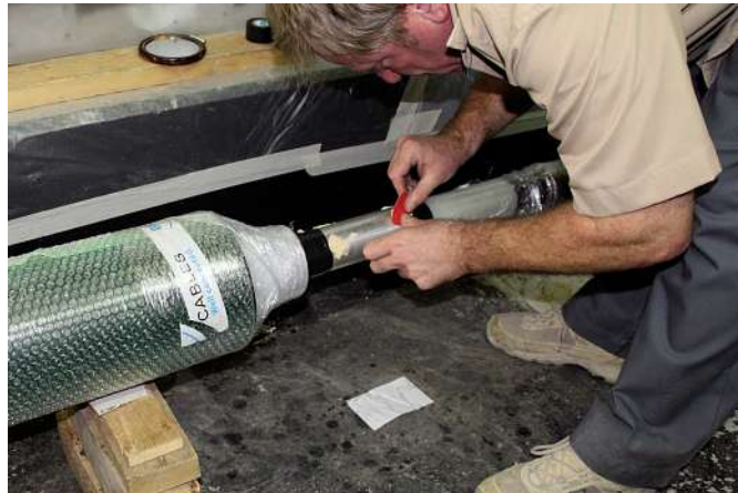
Preparation of the conductor connection for a polymer joint
