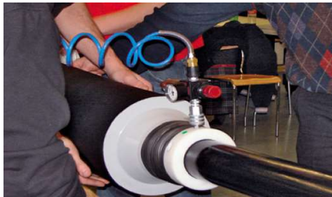
Assembling-friendly installation of a slip-on joint by "air cushion" method
