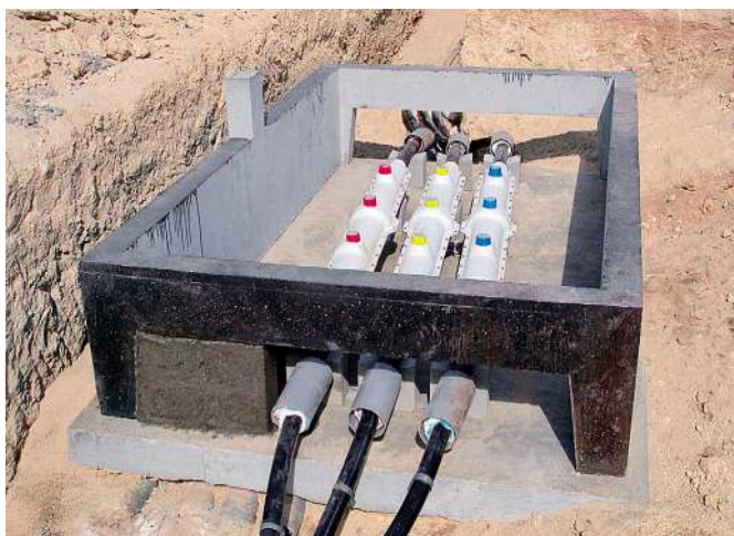
Joints with polyester protection box in a concrete pit
